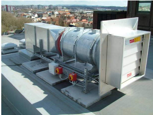
Basic Smoke Control Installation
