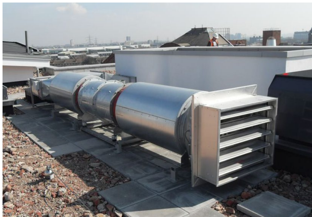
Basic Smoke Control Installation
